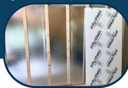
3. Install Poly Shield® with the reflective side facing outward for exterior applications.
