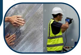
4a. Adhesive attachment: Apply pressure to panel to ensure Poly Shield® is fully adhered. 4b. Mechanical Fasteners: Apply mechanical fasteners to each panel & spacing according to building code requirements
