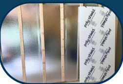
3. Install Poly Shield® with the reflective side facing outward for exterior applications and facing inward towards the living space for interior applications.
