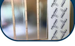
\*R means resistance to Heat Flow. The higher the R-Value, the greater the insulating powe
