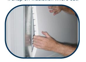
6. Insert the insulation sheet between the horizontal rails.
