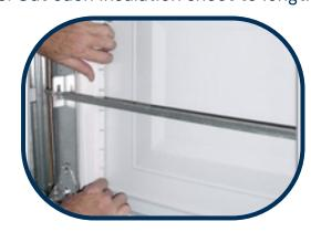
5. Insert the excess insulation behind
