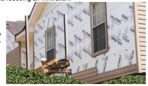
Poly Shield is faced with tough polymeric
